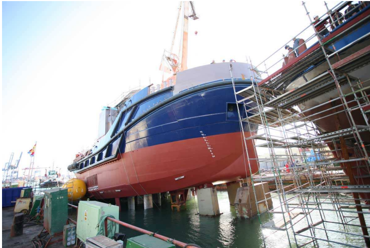
The Solan pictured during construction
